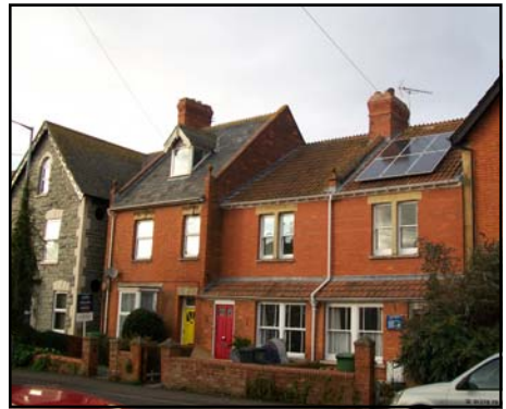
Roof-mounted solar panels are extremely conspicuous within this Glastonbury streetscape
