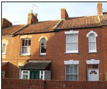
Chimney pots should be retained. Porches should not draw focus away from the host building
